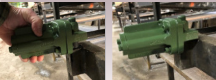
Field Photo of proper installation of female bracket for UH Style Vibrator
